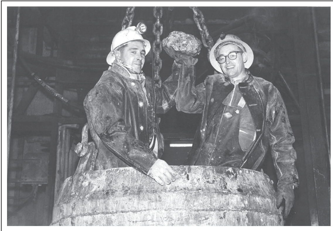
Hitting potash in Esterhazy during the first shaft sinking in 1962.
