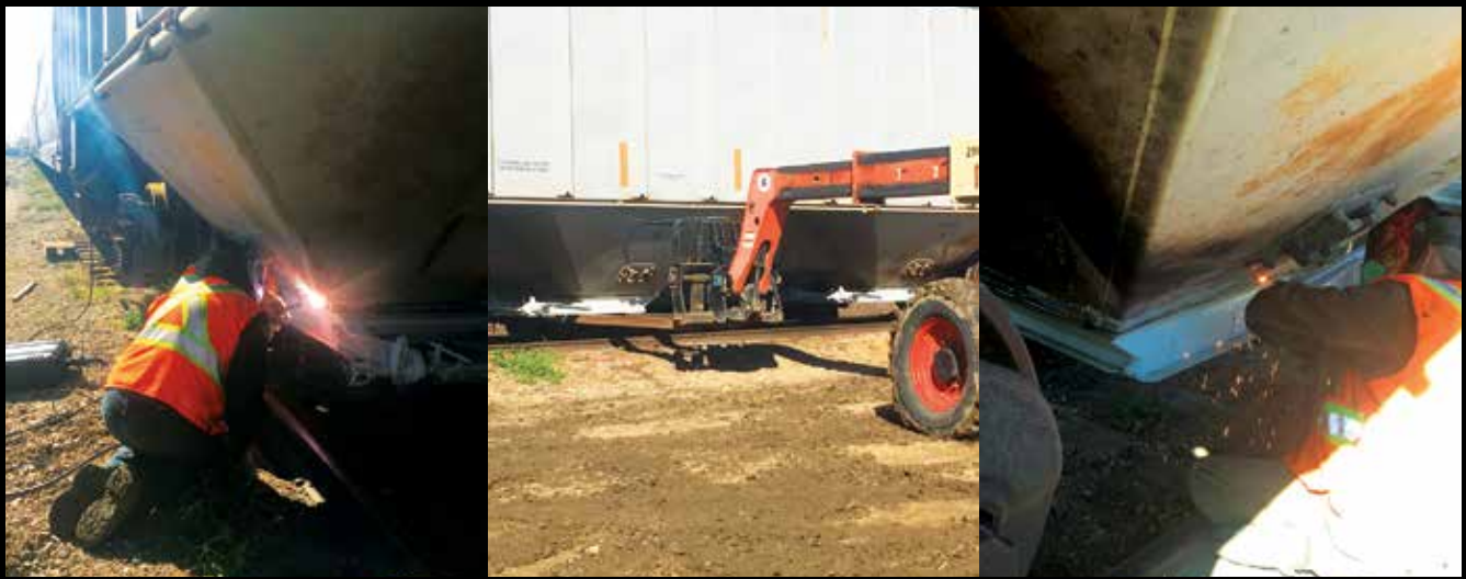
Bottom Outlet Gate Renewal
