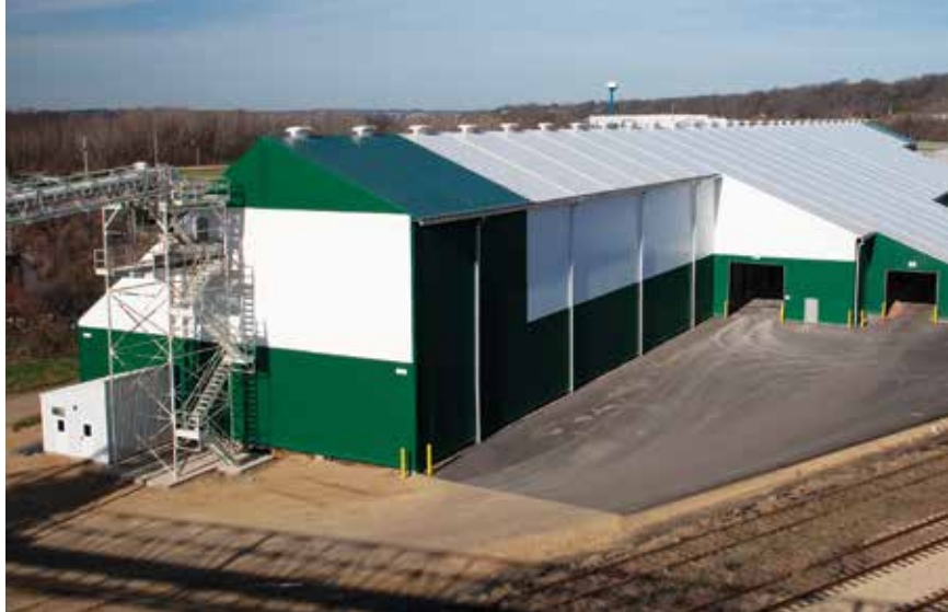
IEI Barge, East Dubuque, IL.
