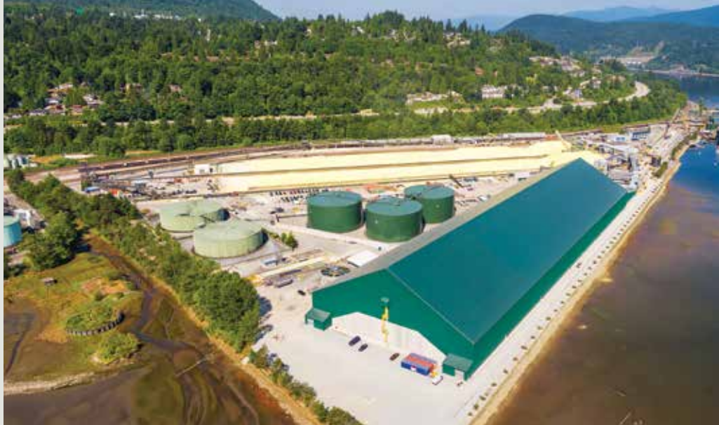
The new potash handling and storage facility in Vancouver port. Front: The 263-metre-long shed for the storage of a total of 160,000 tonnes of potash products. PHOTO COURTESY OF K+S.
